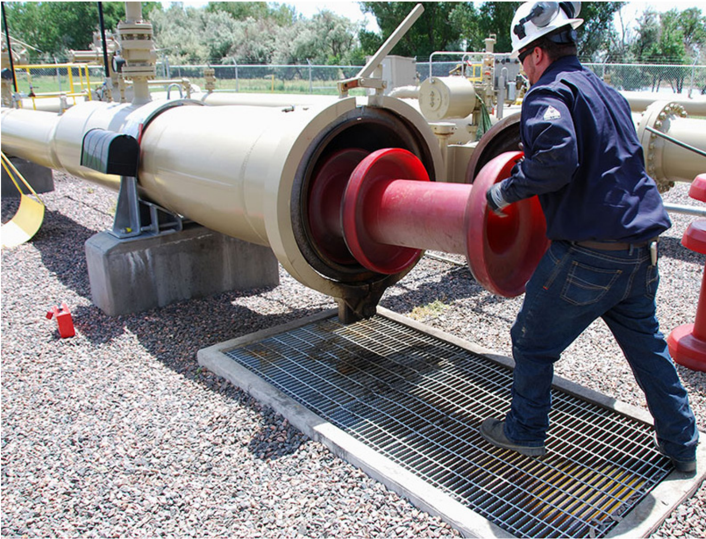
Billy Ops, putting Pig in pipeline
