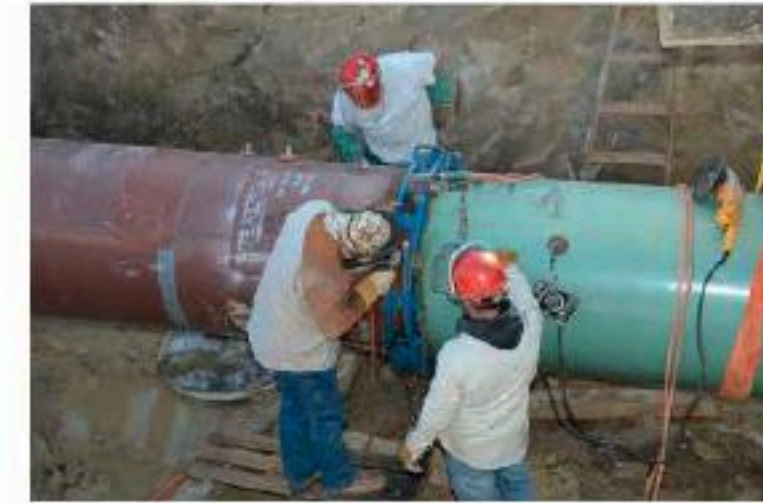
UA Pipefitters work on construction of the Keystone XL Pipeline, AP
